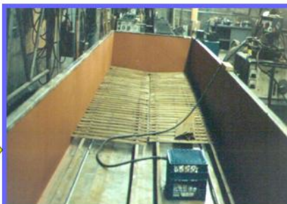
2.- Rebuilding the Vat Interior
